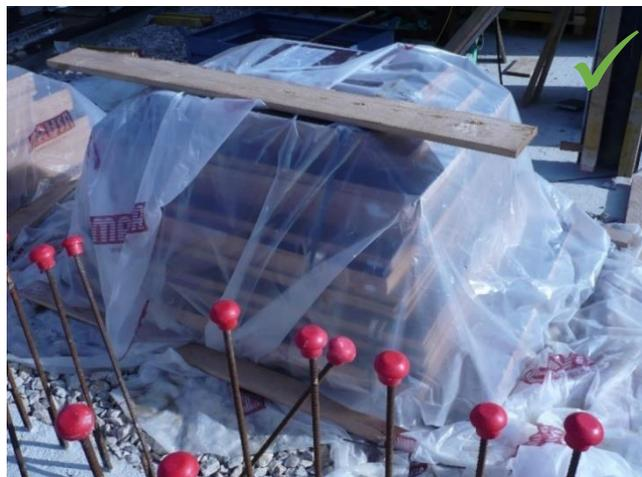
Image 5. Panels protected from a direct outdoors exposure
