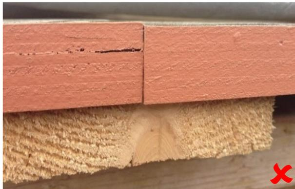
Image 8. Reinforcement, built using untreated wood and failing to keep sufficient gap between panels.
