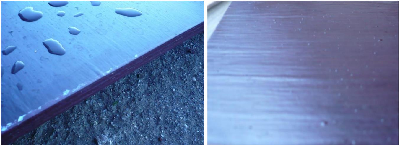
Images. 9 and 10. Typical swelling on the veneers surface due to moisture content variations. “Rippling” effect.
